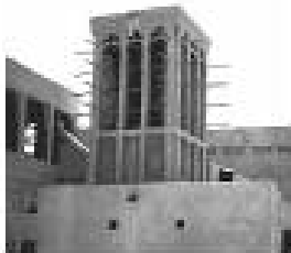
Historical photograph of a wind tower
