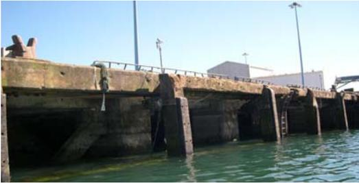
**Photograph of old Dinish Wharf showing evidence of wear and tear on the front face of the structure**
