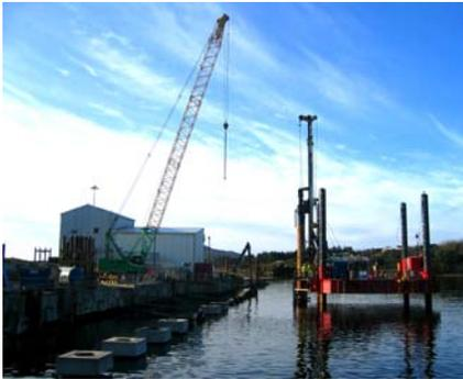
*Dinish wharf replacement at early stage of construction. Precast doughnuts are shown fixed to the cased precast piles*
